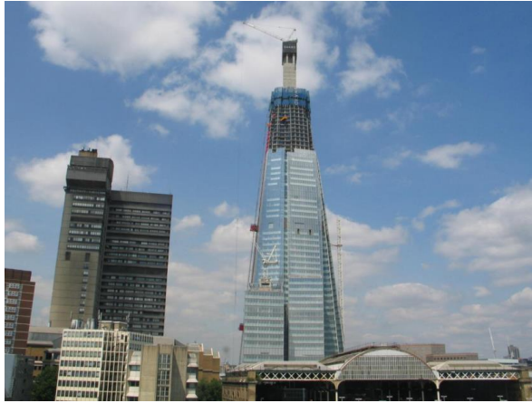
Figure 2. The Shard at London Bridge, showing the interior core during construction.
