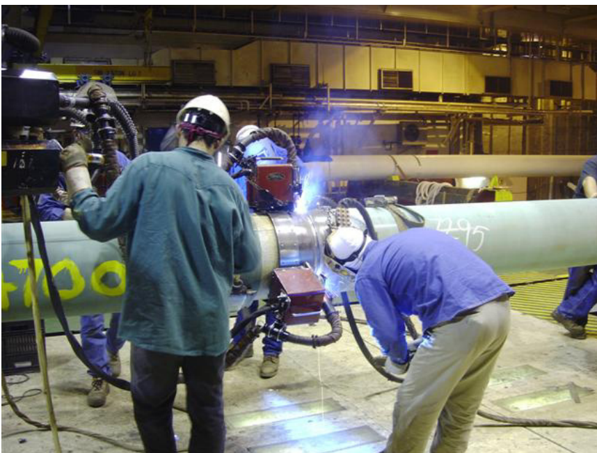
Figure 10. S-lay Welding & NDE Firing Line
