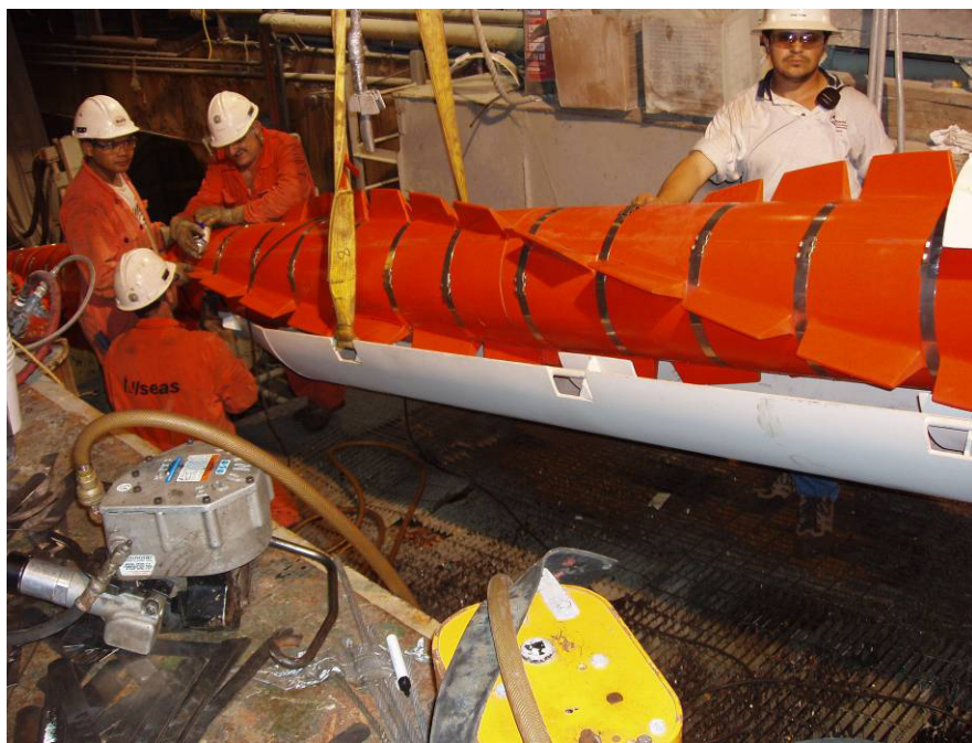
Figure 5. Installation of Helical Strakes on SCR
