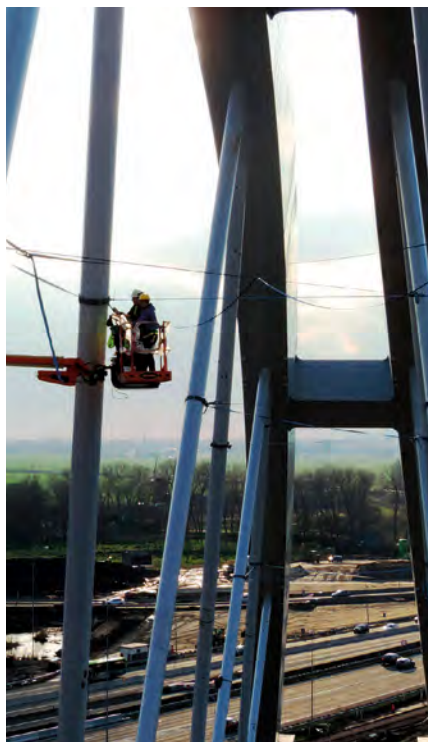
Figure 6 - Assembly of Zandhasen bridge Courtesy: Iv-Infra b.v.
