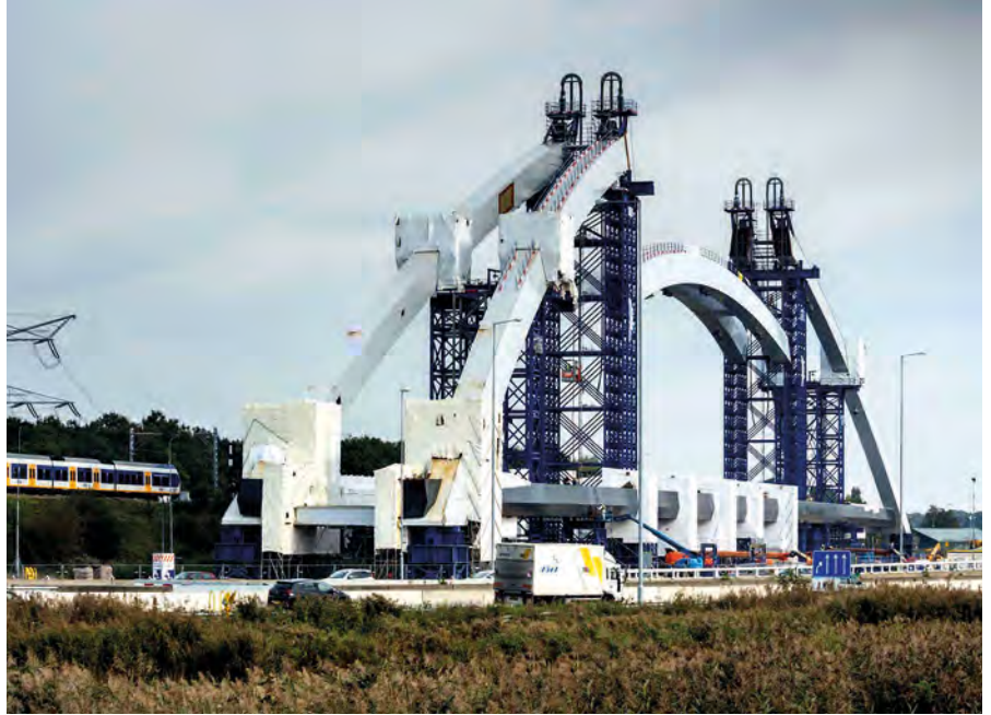
Figure 4 - Assembly of the arch sections using strand jacks Courtesy: Iv-Infra b.v.
