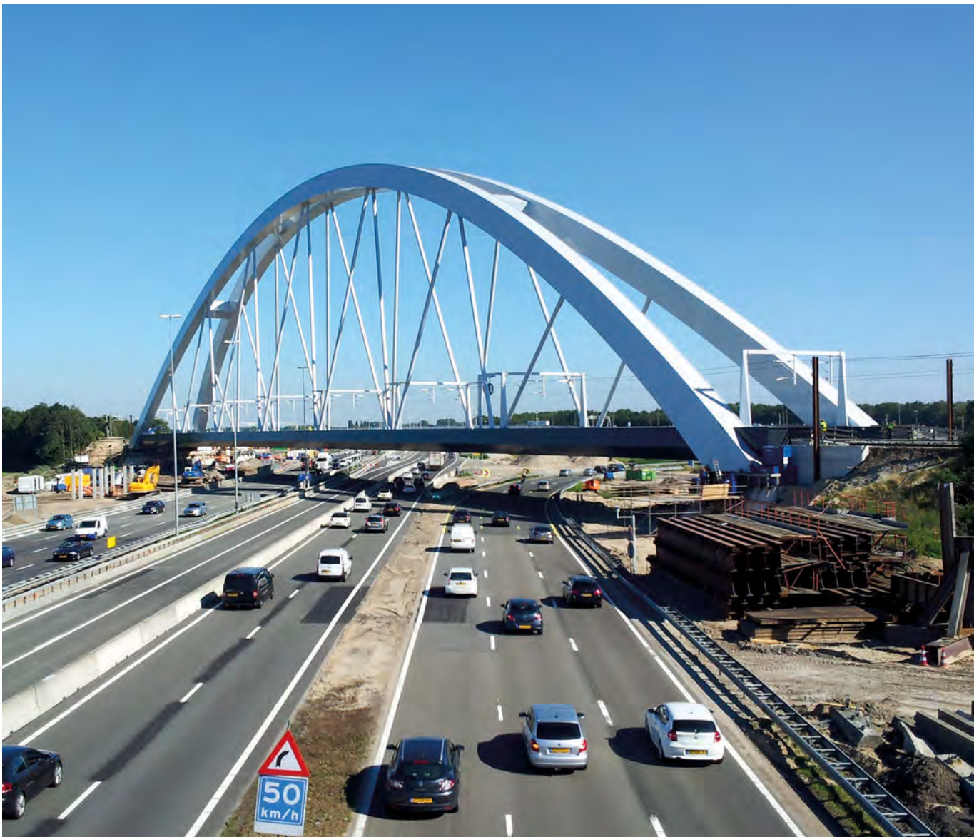
Figure 2 - Zandhasen railway bridge Courtesy: Ronald, licensed under CC BY-SA 4.0
