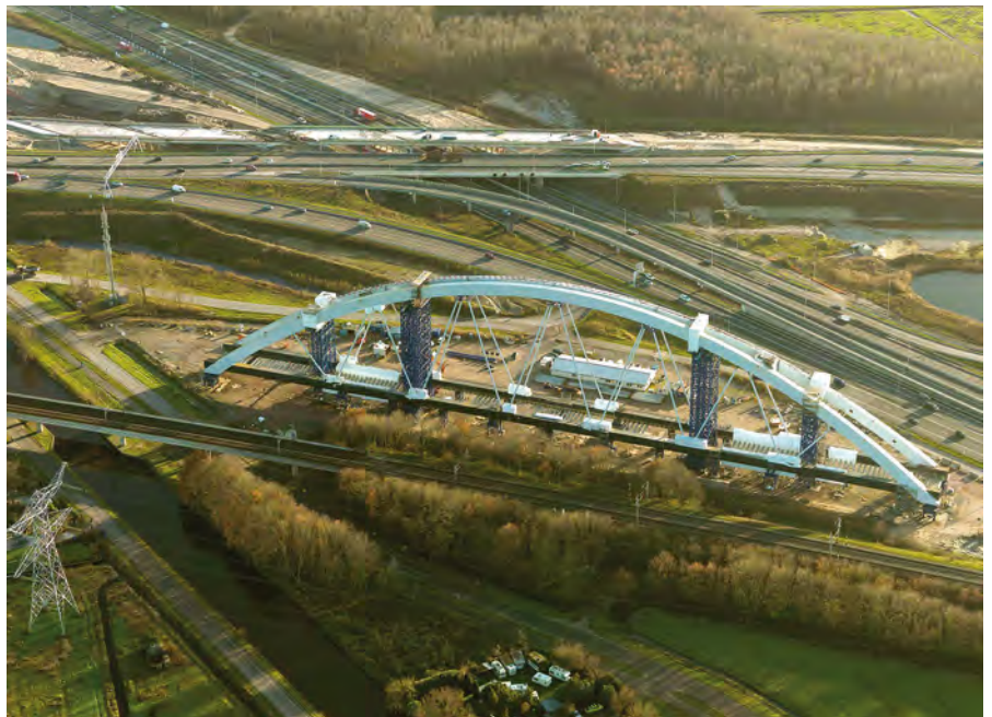
Figure 5 - Assembly of Zandhasen bridge by the side of the A1 Courtesy: Rijkswaterstaat
