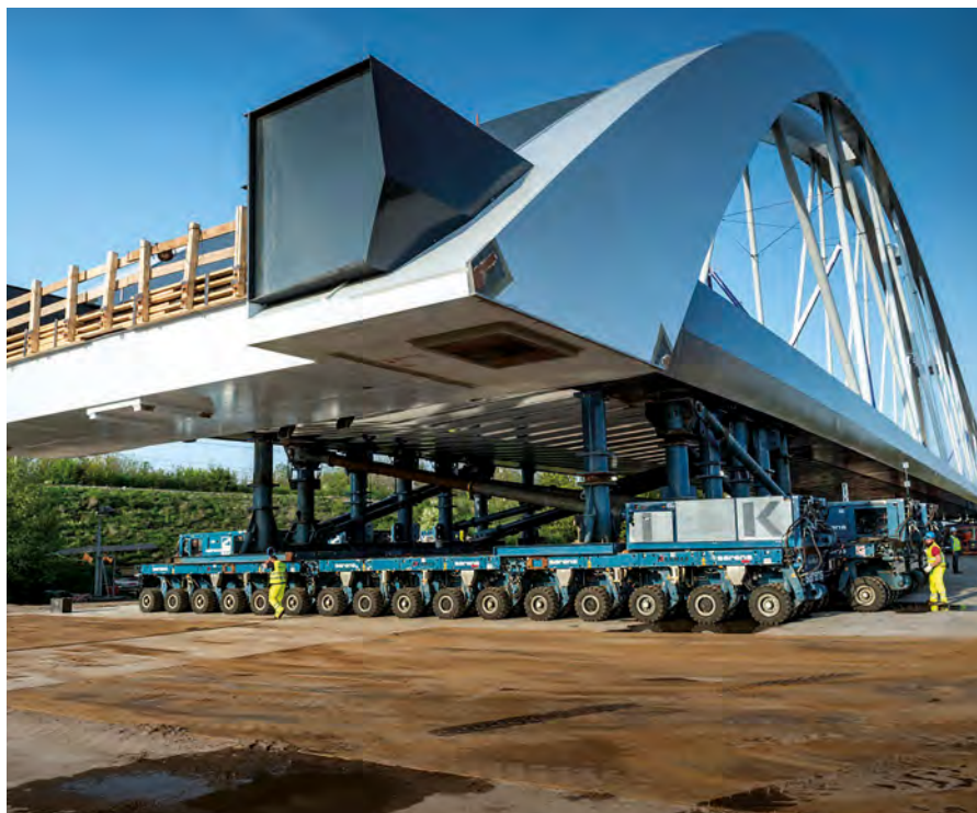
Figure 7 - Bridge being moved over A1 by self propelled modular trailers Courtesy: Iv-Infra b.v.
