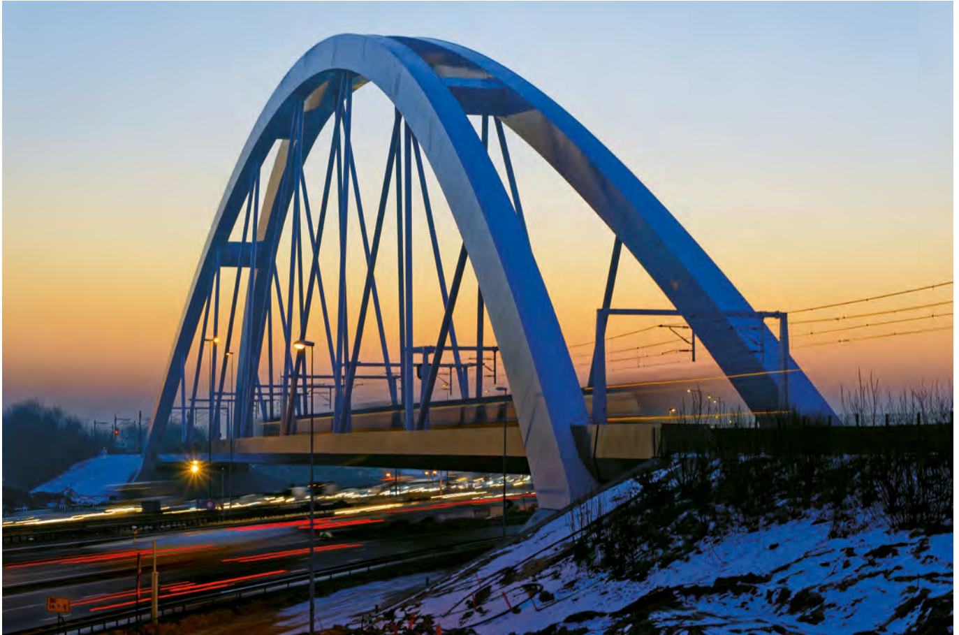
Figure 1 - Zandhazen railway bridge – a tied arch bridge with inclined hangers Courtesy: Iv-Infra b.v.
