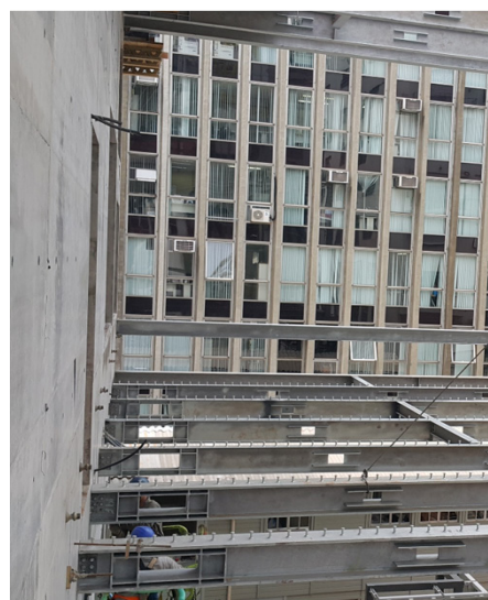
Fig. 10 – The left-side view of the plot and the small space available for work. The right-side assembly of the mixed beams with connection to the metal inserts and to the concrete core Courtesy: José Luiz Canal
