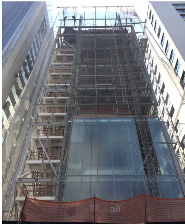
Fig. 12 – Assembly of the glass enclosure system Courtesy: Andrade Morettin Arquitetos Associados
