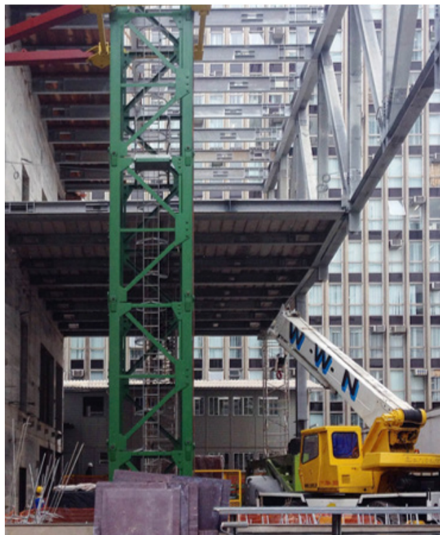
Fig. 11 – Left - hot rolled beams from the floor system of one of the exhibition floors in GR60 steel, with web opening to allow integration of the services. Right - assembly crane, one of the positioned mega trusses, and concrete core Courtesy: José Luiz Canal
