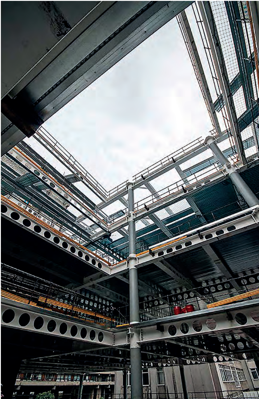
Figure 2 Central atrium and steel framing Courtesy: BCSA
