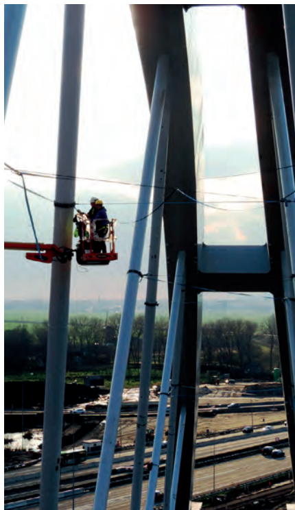
Figure 6 Assembly of Zandhasen bridge Courtesy: Iv-Infra b.v.
