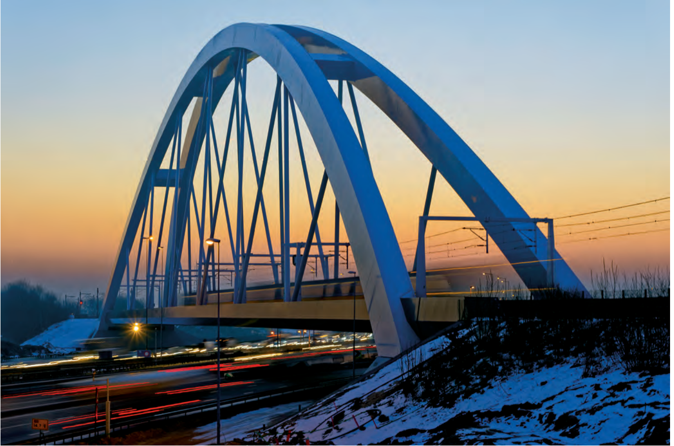
Figure 1 Zandhasen railway bridge – a tied arch bridge with inclined hangers Courtesy: Iv-Infra b.v.
