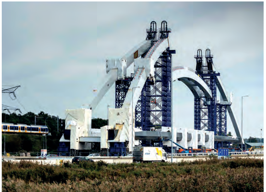
Figure 4 Assembly of the arch sections using strand jacks Courtesy: Iv-Infra b.v.
