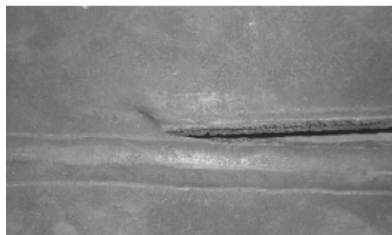
Figure 7. Point at which crack stops in pipe with a diameter of 1220 mm and wall thickness of 17.8 mm fusion line notch location.
