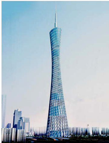
Figure 9. Duangzhou TV Tower
