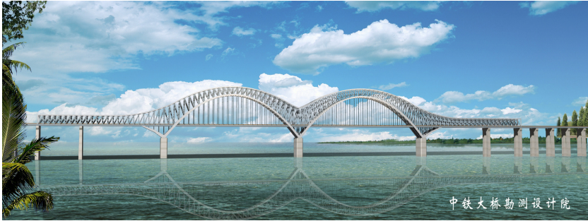
Figure 2. Nanjing Dashengguan Yangtze River Bridge
