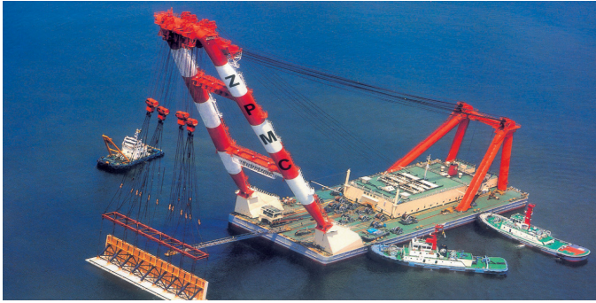
Figure 5. Floating Crane with 4000 tons
