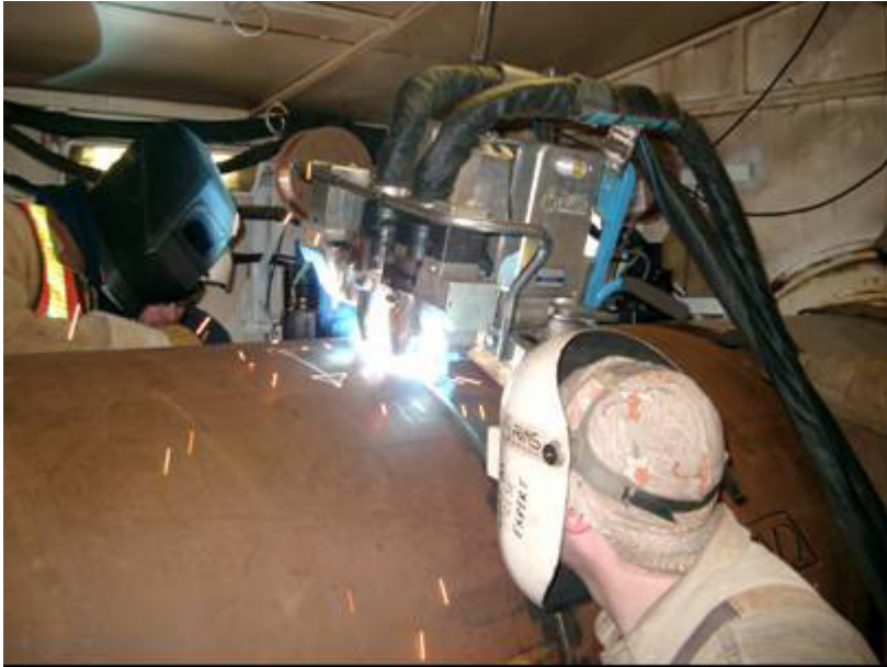
Figure 8. Development of rapid field welding by GMAW for X100
