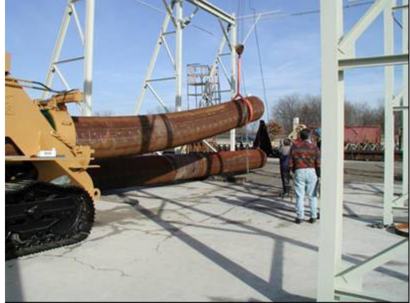
Figure 9. Field bending trials on X100 line-pipe
