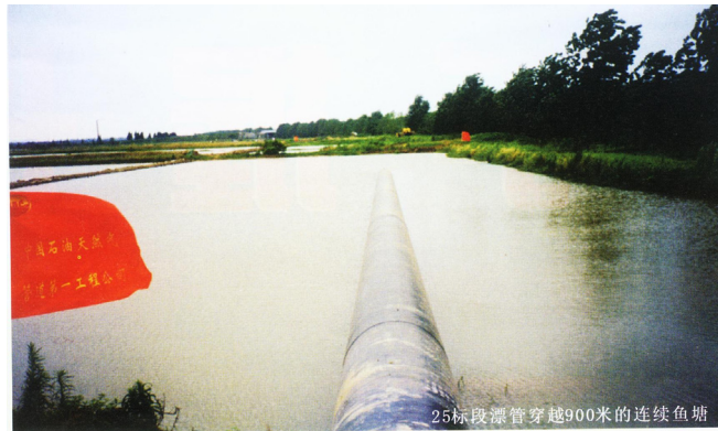
Figure 21. The mooring pipeline traverses the 900 meters swamp in the low and damp region of Eastern China.
