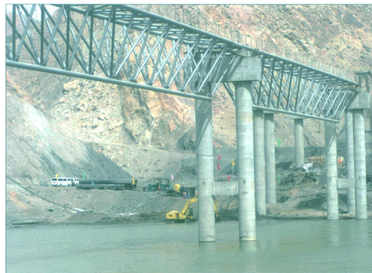
Figure 19. The 540 meter aerial crossing in the upper Yellow River [7].
