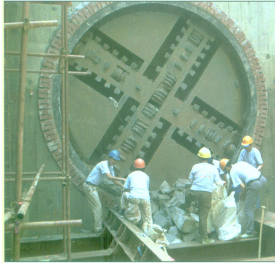
Figure 20. Tunneling machine specially designed for the 1,992 meters long underground crossing of the Yangzi river which is 42 meters beneath the water level and 12 meters under the river bed [7].
