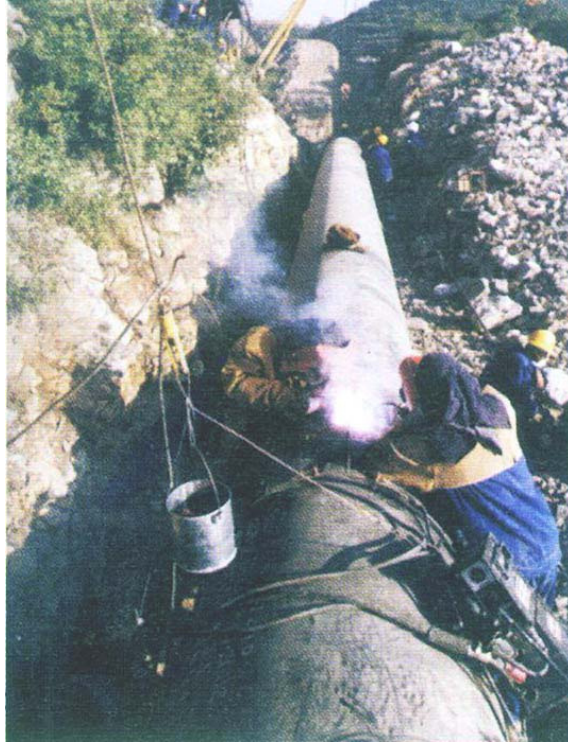
Figure 18. Manual girth welding in a steep terrace
