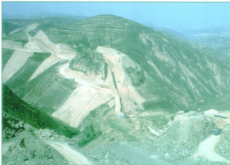
Figure 17. The West- East Gas Project pipeline climbs up the steep hill [7]
