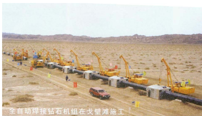
Figure 15. Infield pipe laying and girth welding in the GOBI desert of the West – East Gas Project.
