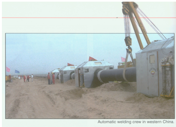
Figure 16. The tests for infield automatic girth welding in the windy and sandy region of the West – Gas Project.
