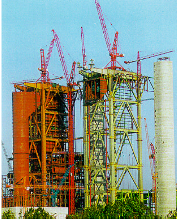
Figure 13: Thermal power station Schwarze Pumpe, Germany.
