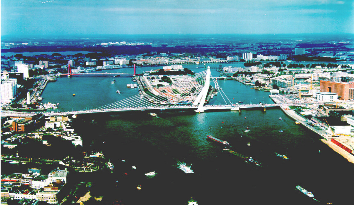
Figure 16: Bridgebuilding with heavy plates, Erasmus-bridge, NL.
