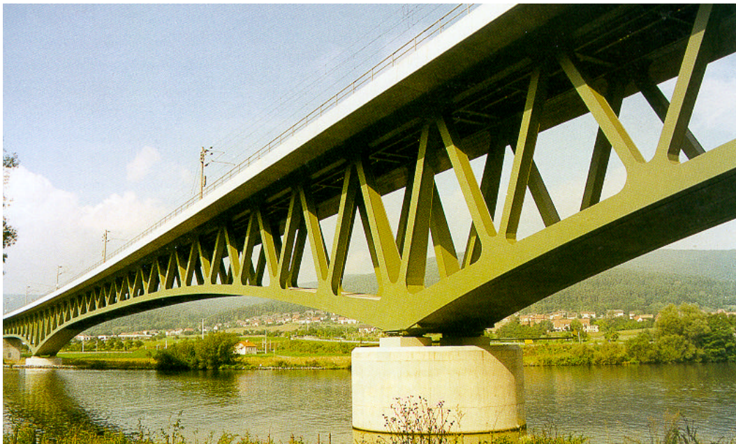
Figure 15: Bridgebuilding with heavy plates, Nantenbachtal-bridge, Germany.
