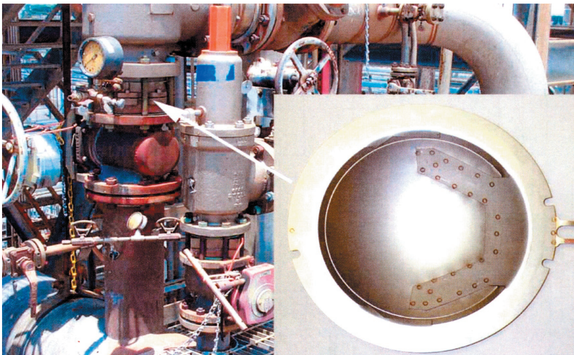
Figure 1: A 46 cm diameter niobium rupture disk installed in a vapor line of an acetic acid drying column.
