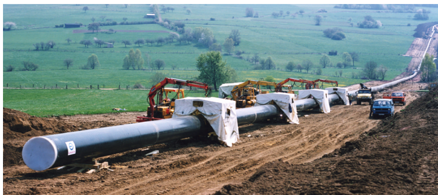
Figure 3: X80 pipeline construction in Germany. Courtesy of Europeipe.
