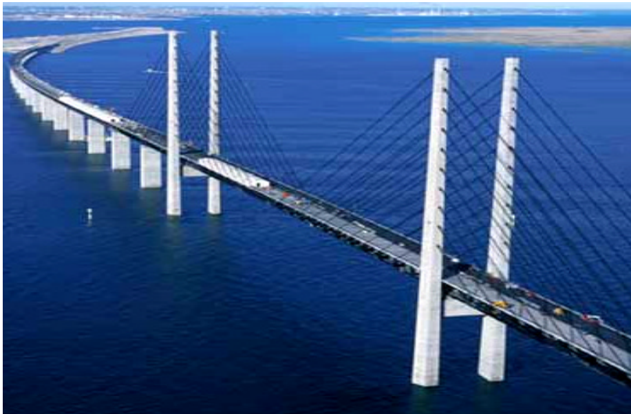
Figure 10: The Öresund Bridge.
