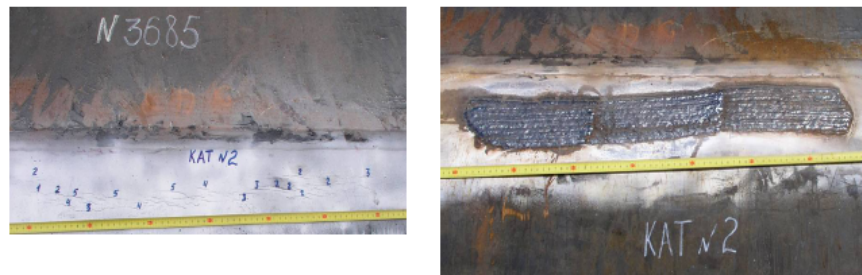
Figure 8. Development of fitness criteria for repair and technology of SCC defects using repair welding
