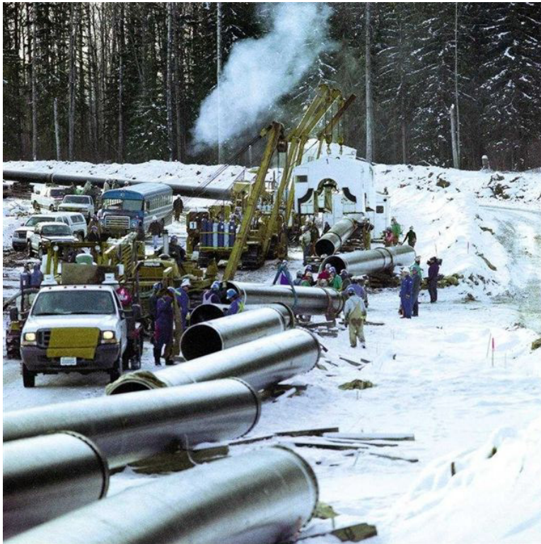
Figure 7. Winter construction of Godin Lake X100 project
