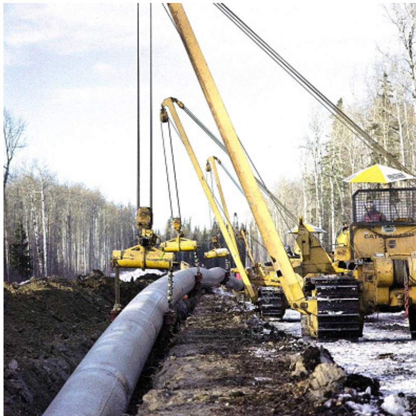
Figure 10. Lowering-in of X100 on Godin Lake
