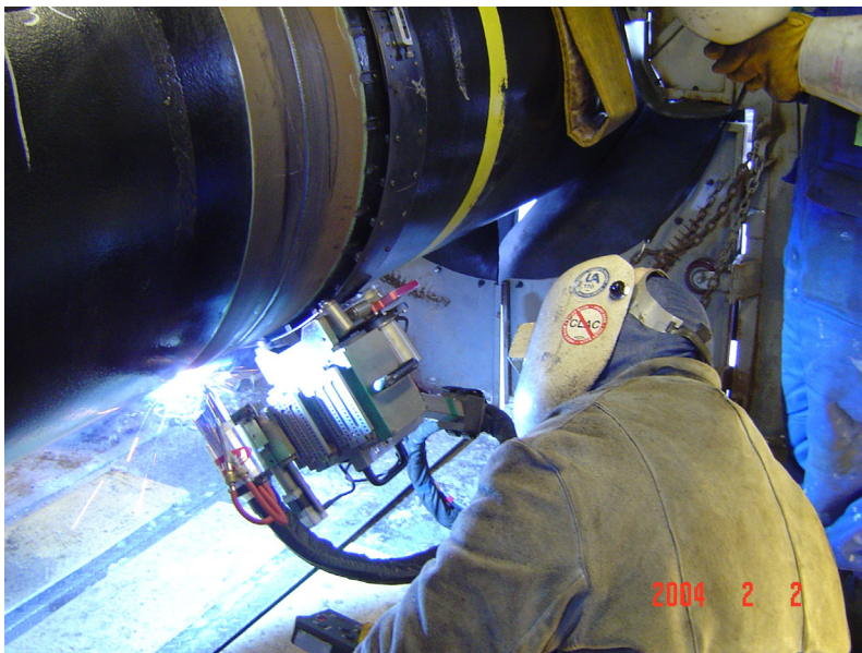
Figure 8. Application of single tandem on welding X100 Godin Lake
