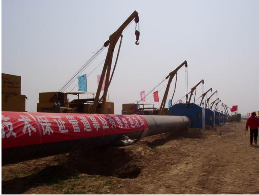
Figure 3.11 1016mm diameter X80 line pipes being laid in the Ji-Ning pipeline project
