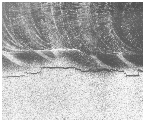
Figure 2. Lamellar tearing in a T-joint weld, source TWI [9].
