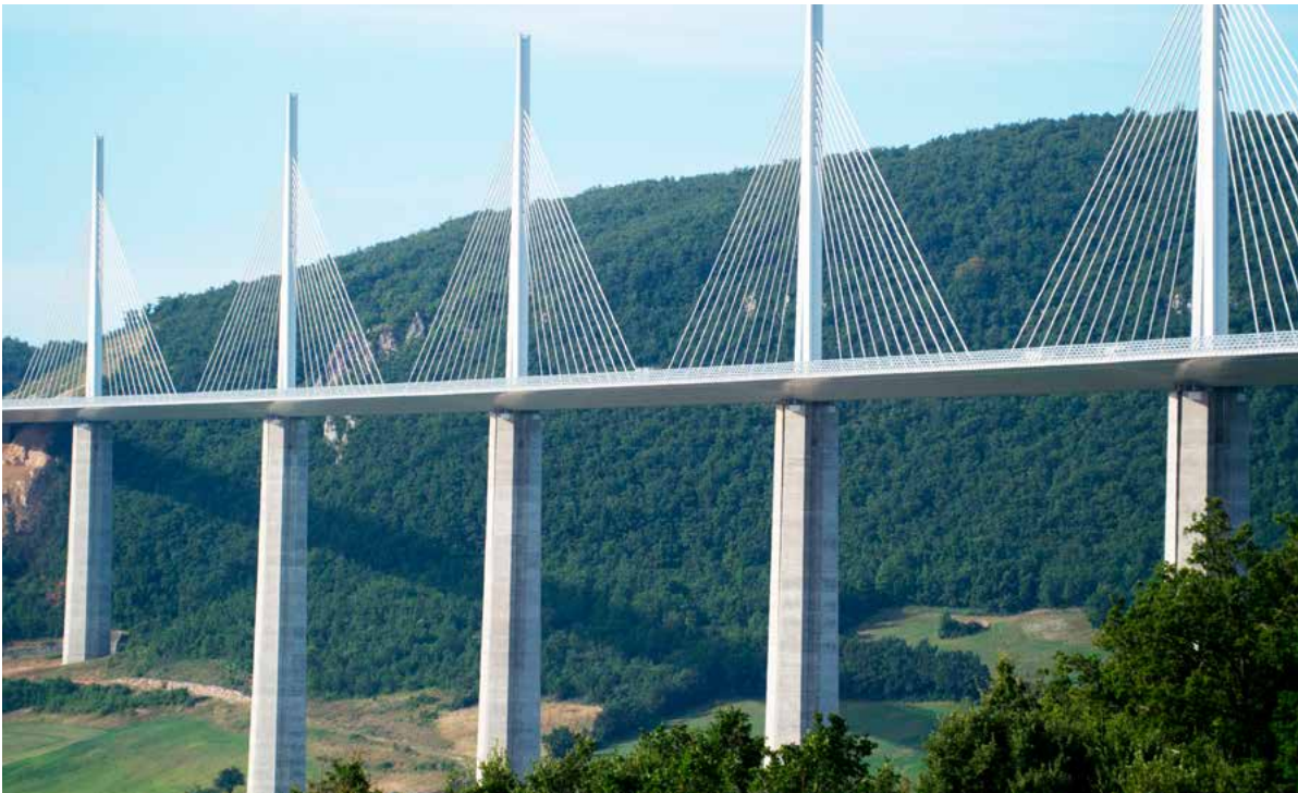
The Viaduct de Millau bridge in southern France stands as the tallest bridge in the world at 343 m (1,125 ft). Niobium was used at the rate of 0.025% per tonne of steel to reduce its overall weight by some 60 percent.
