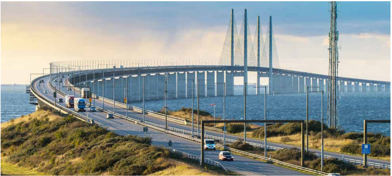
Øresund Bridge connects Denmark and Sweden and was constructed with 82,000 tonne of high strength steel. With a 0.02% Nb addition, a 15,000 tonne reduction in weight and a cost savings of $25 million were realized.
