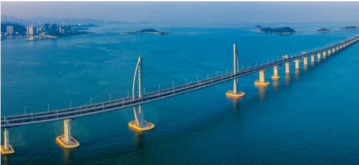
The Hong Kong- Zhuhai-Macao bridge is the world's longest cross-sea project at 55Km (34 miles), incorporating a bridge and a 6.7Km (4 miles) seabed tunnel. The HBIS Group optimized levels of vanadium, chrome, niobium and copper to provide high strength, anti-seismic wire bars with an unprecedented anti-corrosion ability used for the immersed tunnel construction.
