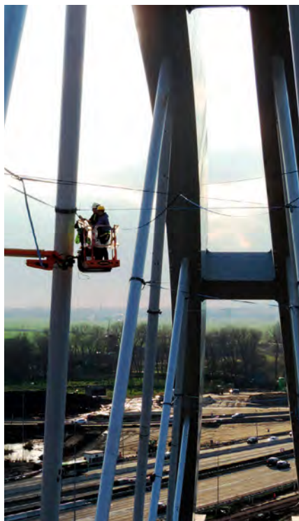
图6 组装Zandhazen 桥 资料来源: Iv-Infra b. v.
